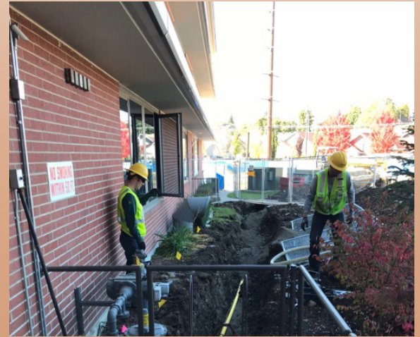
New gas line is being installed to to the Terrace building
