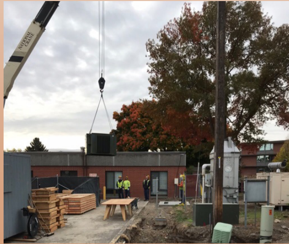
Avista crew setting the new transformer
