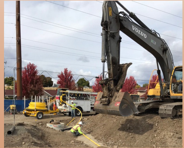
Lance Pounder bedding gas line with sand
