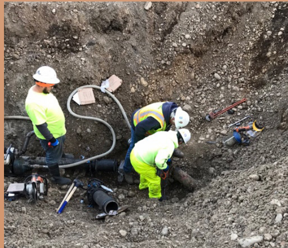
Lance Pounder crew make new sewer line tie-in
