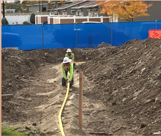
Avista crew installing new gas line
