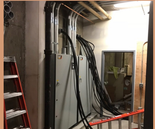
Summit Electric pulled in new wires for the generator power
