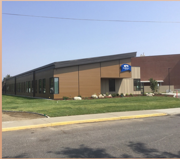
Completed landscaping on West side
