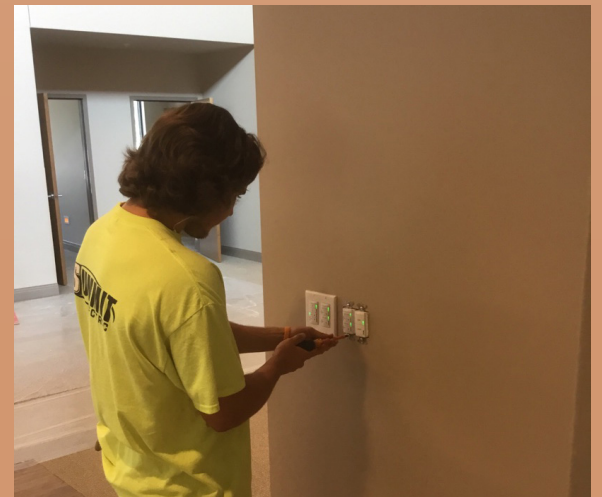
Summit Electric installing electrical trim plates
