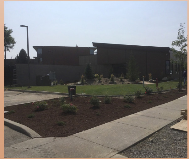
Landscaping is completed on the East end
