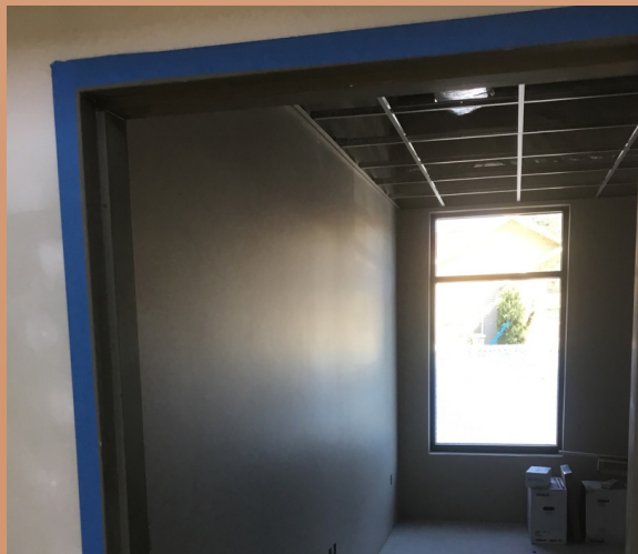
LAC Drywall has done a fine job taping and finishing walls
