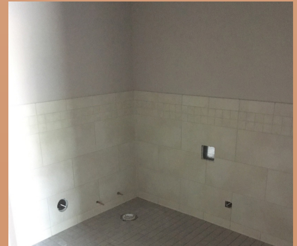
Ibex Flooring continues to do a great job installing resident bathrooms
