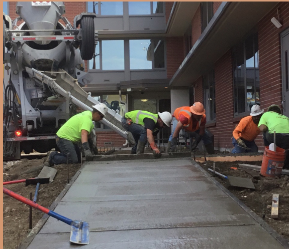
Five Star Concrete pouring and finishing sidewalks in the inner courtyard
