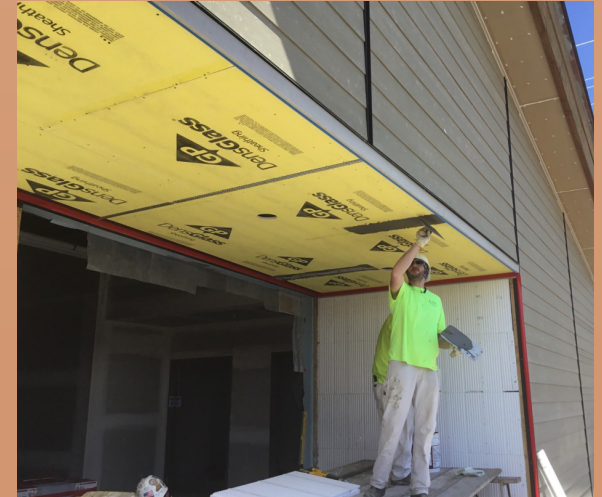
LAC Drywall applying EIFS to soffits
