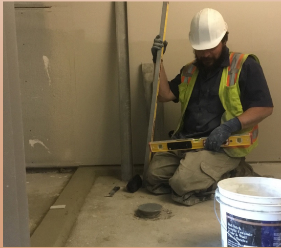
Ibex Flooring setting mortar beds in the resident room bathrooms
