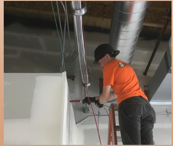
Summit Electric pulling fire alarm wiring above ceiling
