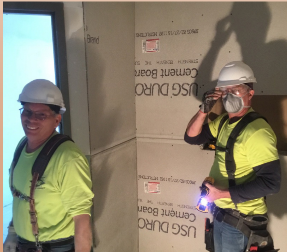
LAC Drywall installing cement board in the showers for tile
