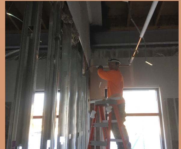
Specialty Insulation insulating water piping
