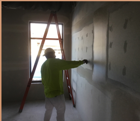
LAC Drywall is taping and finished resident rooms in Zone 2
