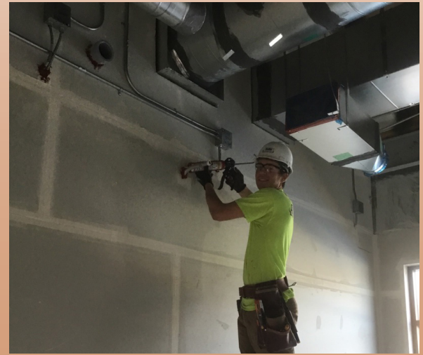
Summit Electric is fire caulking above-ceiling in Zone 2
