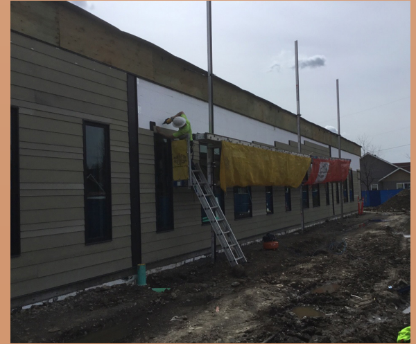
Riverside Exteriors is installing lap siding on the North elevation
