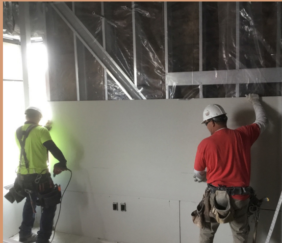
LAC Drywall hanging drywall in resident rooms
