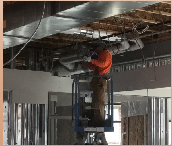
Apollo Mechanical roughing-in duct work above ceiling
