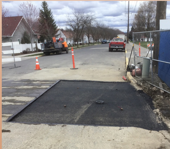
Lance Pounder Excavating paved where the sewer main tap occurred
