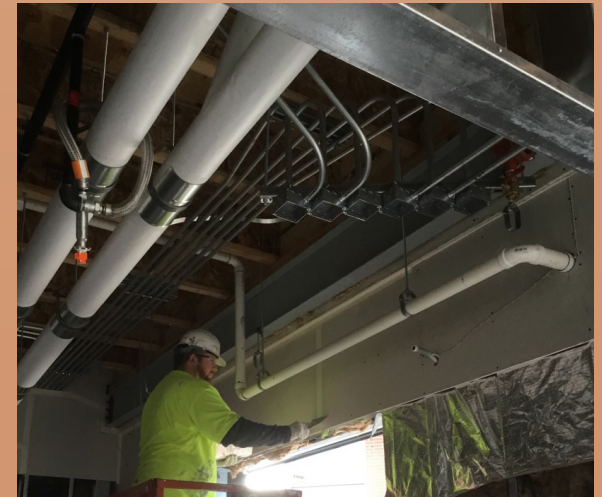
LAC Drywall fire taping above-ceiling
