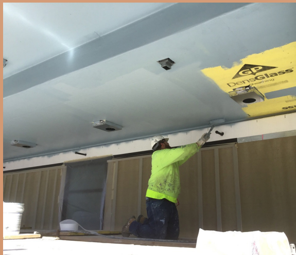
LAC Drywall applying fluid weather barrier to soffit
