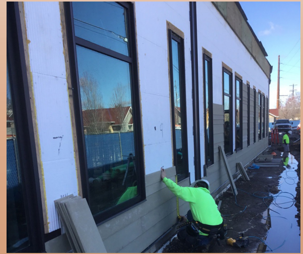
Riverside Exteriors installed lap side on the North elevation
