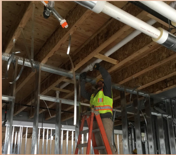
KC Charles roughing-in vent lines above ceiling
