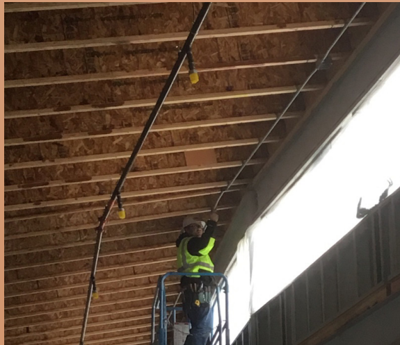
Summit Electric roughing-in conduit above ceiling
