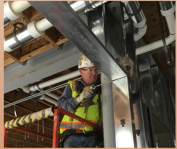
LAC Drywall framing interior walls
