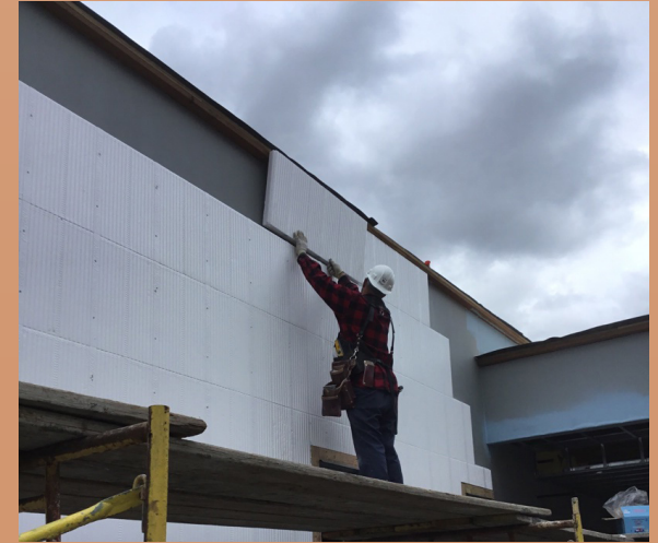
LAC Drywall installing InSoFast insulation to exterior walls
